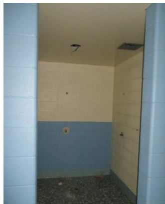
Photo: Fixtures Removed
