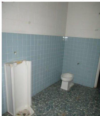
Photo: Fixtures Removed
