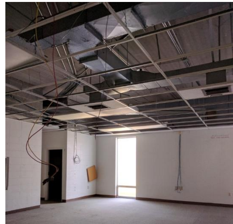
Photo: Typical semi-demolished space
