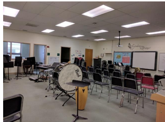
Photo: Typical Classroom Lighting
