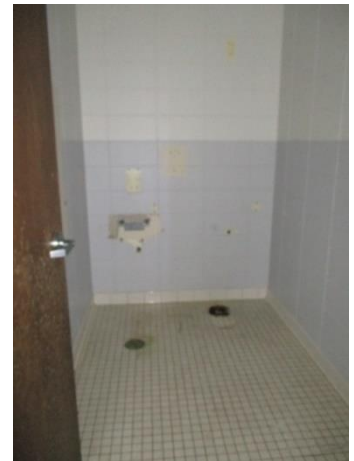
Photo: Fixtures Removed
