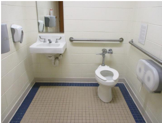
Photo: ADA Floor Mounted Water Closet
