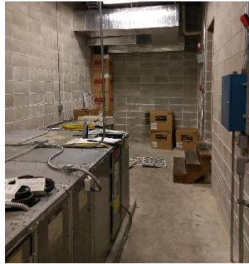
Photo: Indoor AHU DX Unit Photo: Indoor AHU DX Unit
