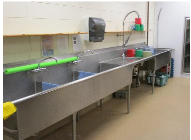
Photo: Three Compartment Sink
