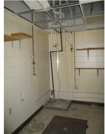
Photo: Water Heater Removed
