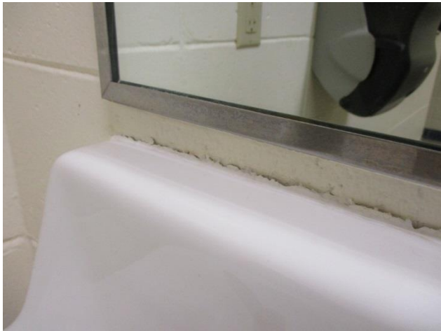
Photo: Recalk Fixtures
