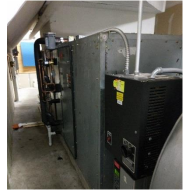
Photo: Indoor AHU DX Unit Photo: Indoor AHU DX Unit
