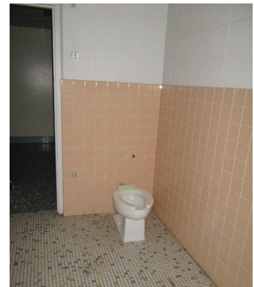
Photo: Fixture Removed
